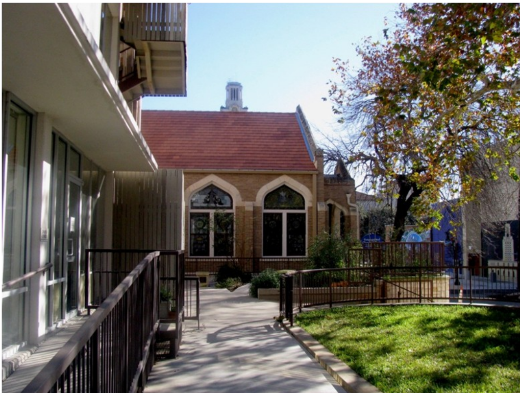
The church on Dec. 27, 2009—our new access to the sanctuary and to the Towery wing from San Antonio St.—there are still steps from 23rd St.
