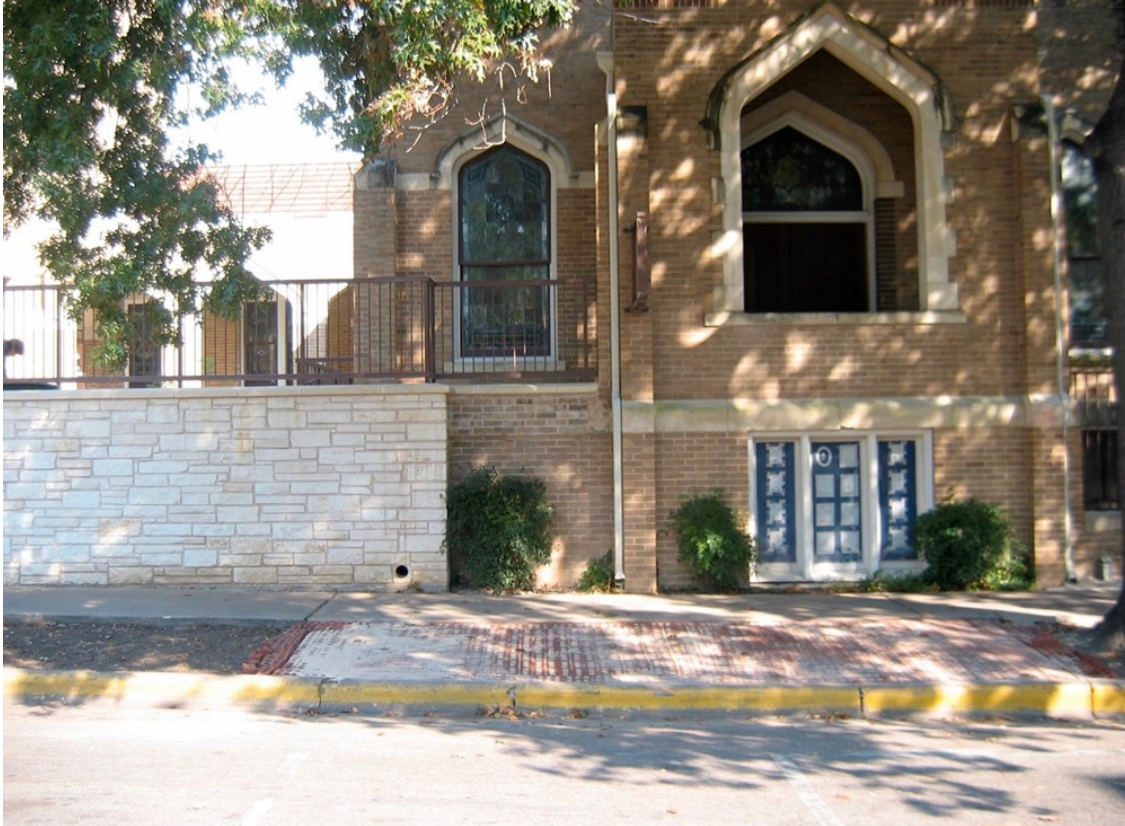
11/4/07 New front of the church—note that the stairs into the sanctuary are no longer there
